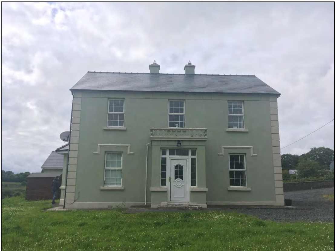
Plate 4-12 Dwelling house in Kileerreen, to be demolished.
