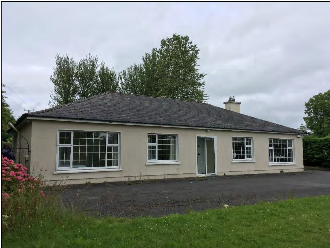
Plate 4-2 Dwelling house to be demolished at Gortaloura, classified as Buildings and Artificial Surfaces (BL3)
